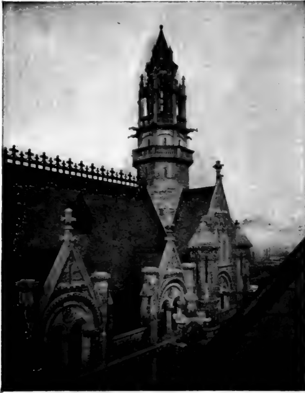
THE PRUDENTIAL TOWER.
